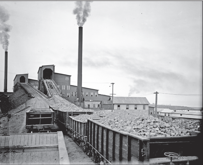
ROCK--A line of carts carrying copper-rich rock wait to move into a stamp mill for the Mohawk and Wolverine mines, where the rock was crushed. Photo courtesy of Michigan Technological University Archives and Copper Country Historical Collections)
